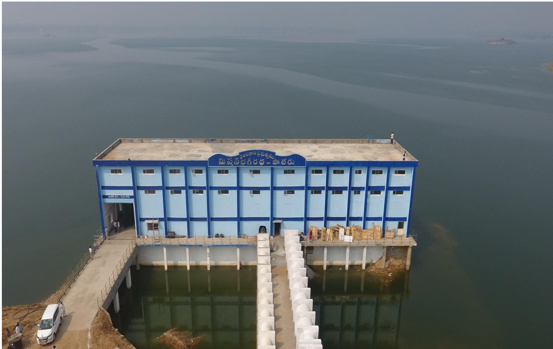
55m x 12m x 14m Intake well
