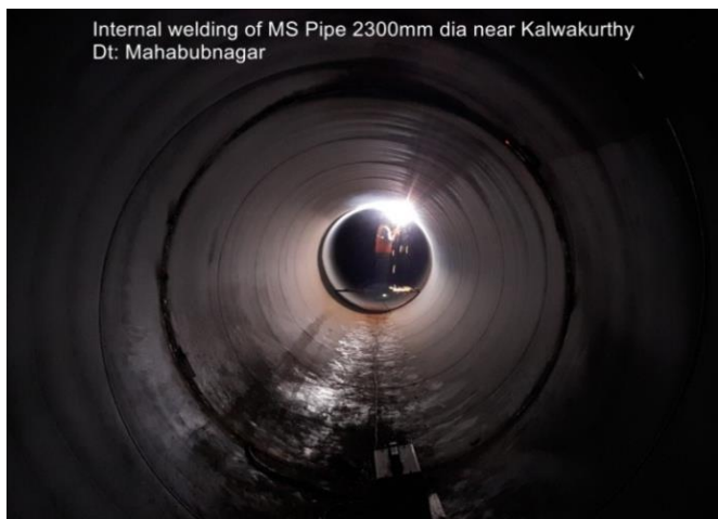
2.4 mtrs dia MS Pipe line
