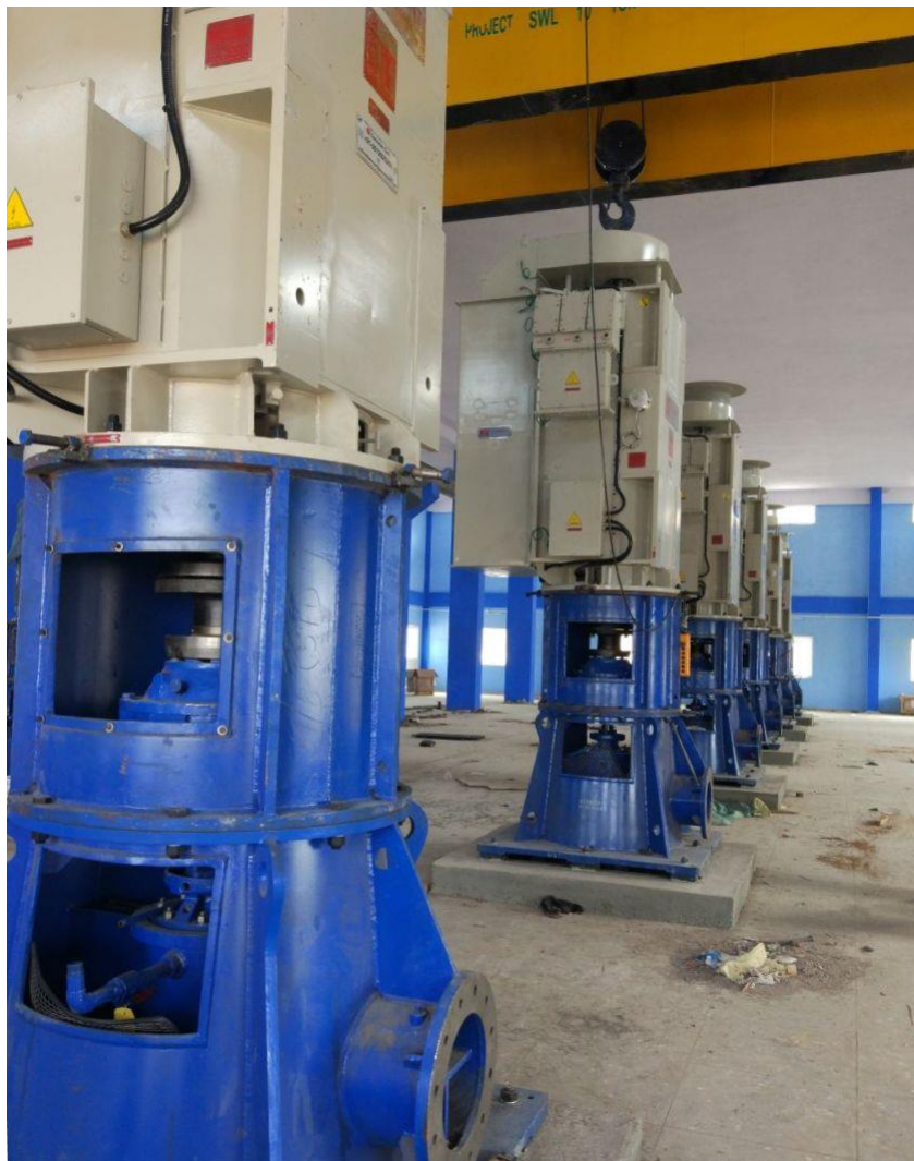
Pumpsets @ Mallannagutta WTP
