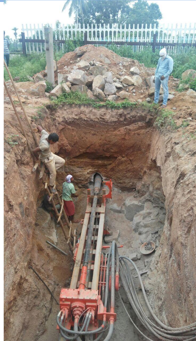
Railway crossing @ Vangapally
